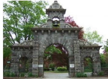
Lawrence Street Gate/Office
